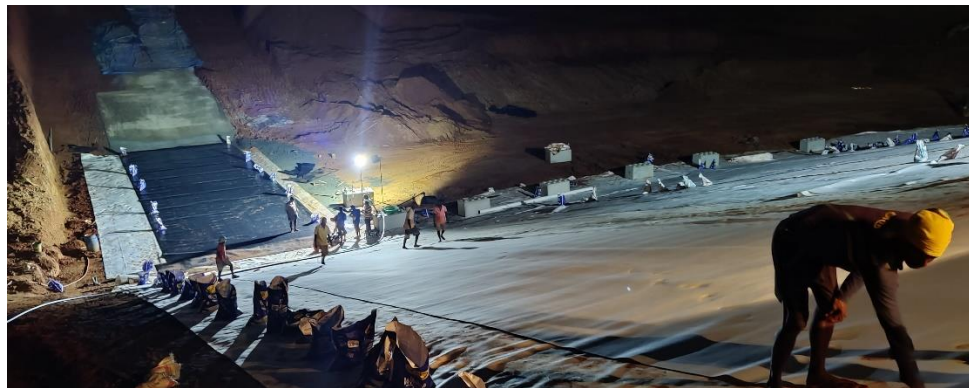
Figure 24: Waterproofing of the Wall Foundation
