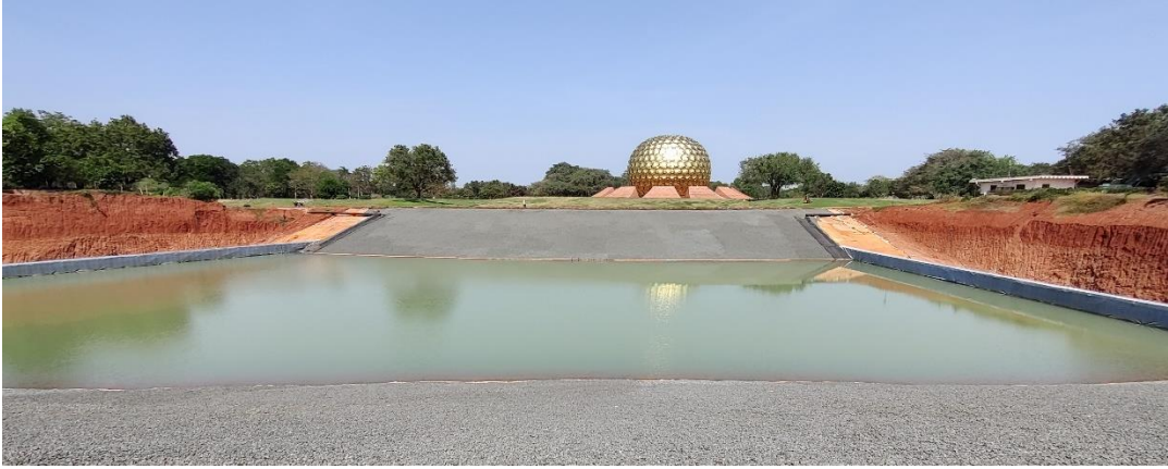
Figure 25: Water level at 7.5m & Concrete Block Wall at 10m
