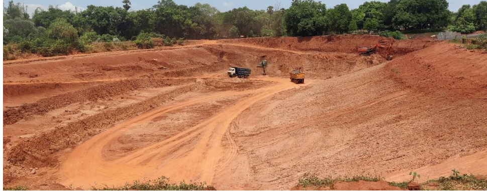
Figure 23: Excavation of lake section
